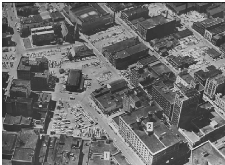
An aerial view of the Midtown site, looking south from East Avenue, taken before construction began.
