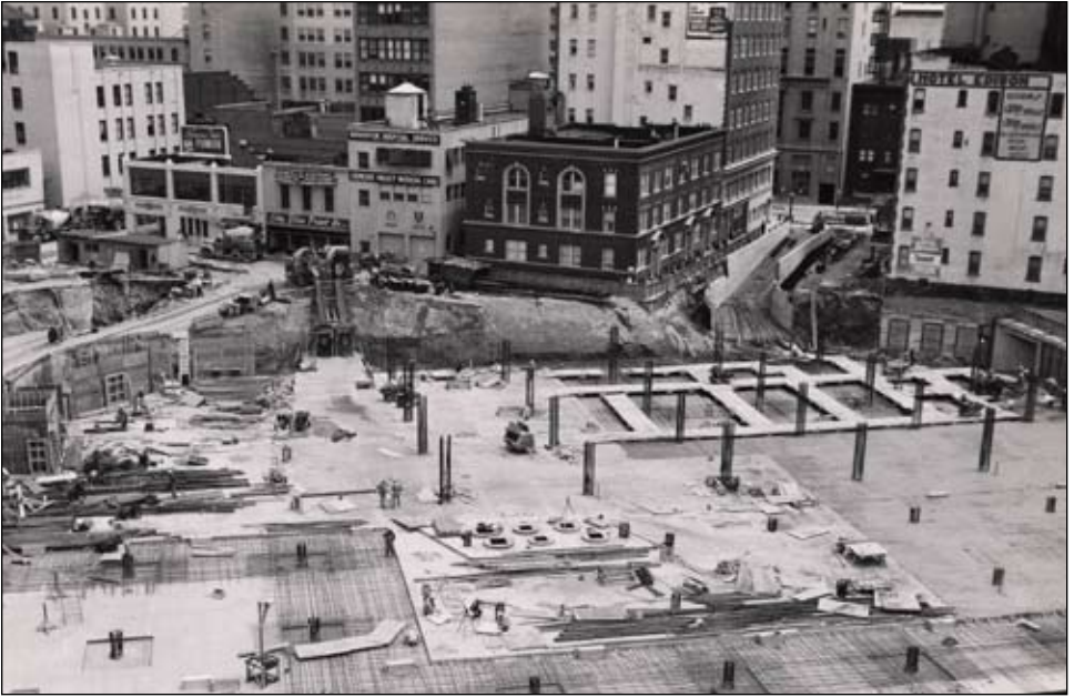
Ground was broken on April 6, 1959. This image, taken in Spring 1961, shows construction of the underground garage.
