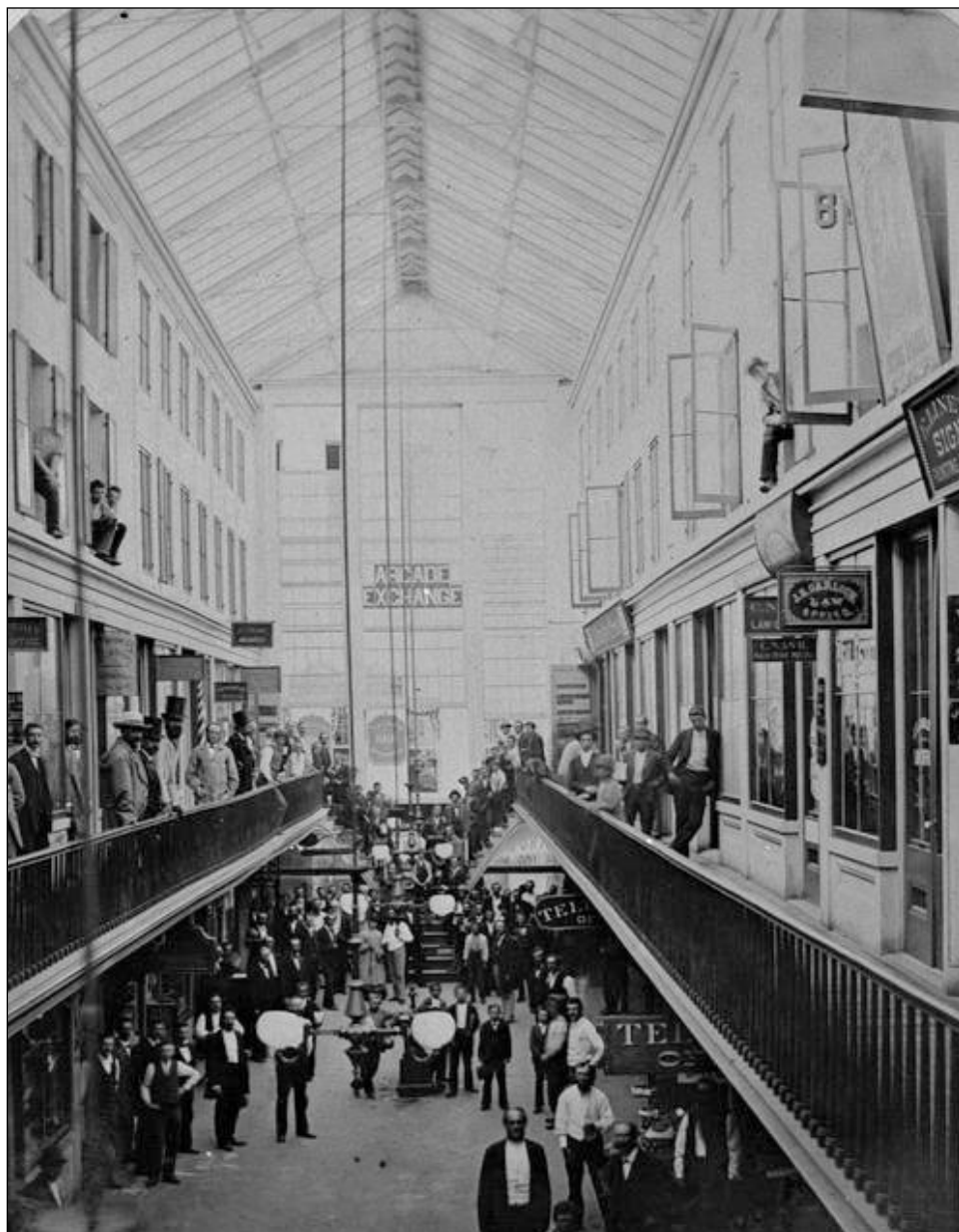
The vision Victor Gruen proposed was more similar to Rochester's historic Reynolds Arcade than to an enclosed shopping mall. The Arcade, first built in 1828, was the dream project of Abelard Reynolds, a pioneer settler of Rochester. The original Arcade building, which stood until 1932, was the focal point of the city. It had everything: the post office, John Bausch's optics shop, Western Union Telegraph, a library and meeting room, and a variety of shops carrying everyday and luxury goods. Photograph courtesy of Rochester Public Library, Local History Division.
